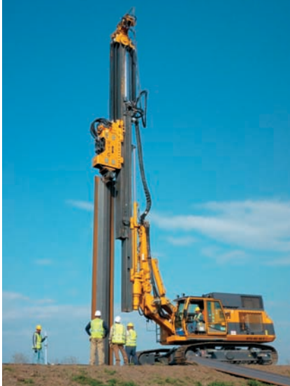
Vibrationsrammung Driving with Vibrohammers
