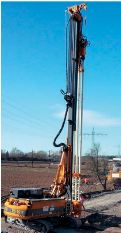
SMW Soil Mixing Wall
